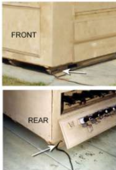
Figure 5.17. Grounding Locations on the PDC.
