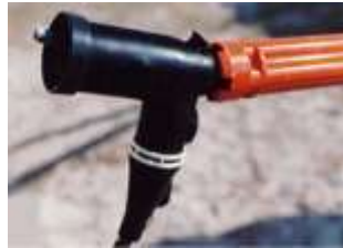
Figure 2.12. Load Break Elbow (secured with Grip-All clamp stick).
