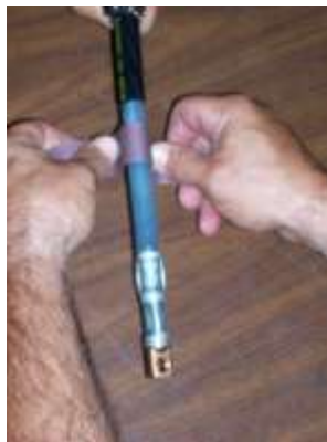
Figure A2.15. Cleaning Insulation with Abrasive Cloth.
