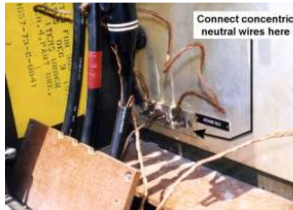
Figure 4.13. SDC Input Ground Connection.
