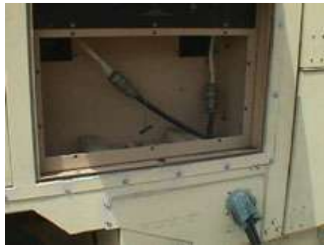
Figure 5.30. Control Cables Connected at MEP-12A.
