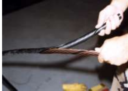
Figure A2.3. Stripping Away Cable Jacket.
