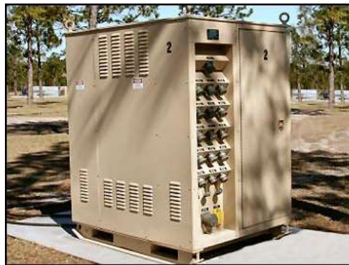
Figure 2.3. Secondary Distribution Center (SDC), Low-Voltage Side.
