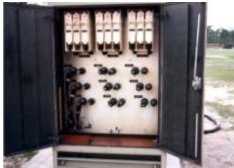
Figure 4.14. Cables Connected to Input Bushings.
