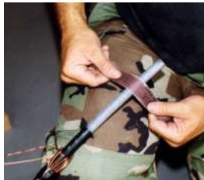
Figure A2.7. Sand and Clean the Insulation to Remove Marring.
