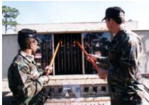
Figure 5.26. Disconnecting the Arc Strangler Switches.
