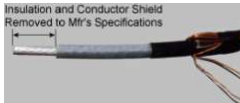
Figure A2.8. Remove Insulation from Conductor.
